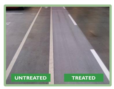
Many concrete floors are installed with a highly polished finish. This creates a very serious risk of slipping when the surface becomes wet.
